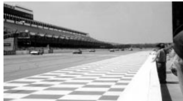
The scale of the raceway is imposing with very solid concrete walls surrounding the oval section.
